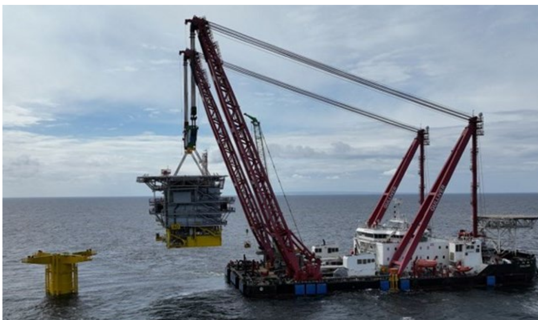
Figure 54: Substation installation vessels 95
